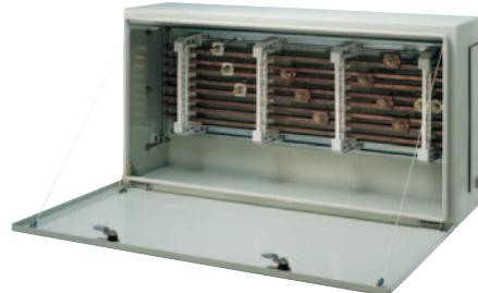
cable and conductor entries to suit the user's requirements, but without exceeding the certified maximum number.
